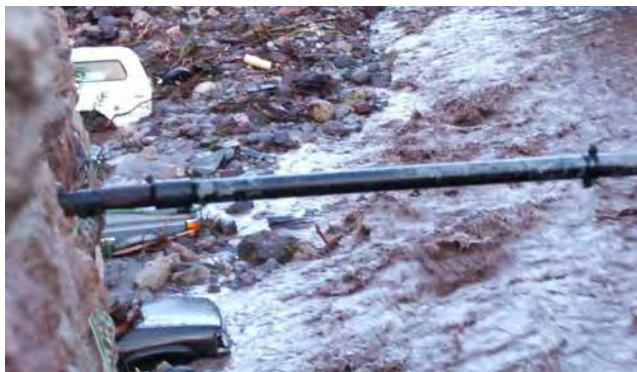
2013 flooding in Mogollon
